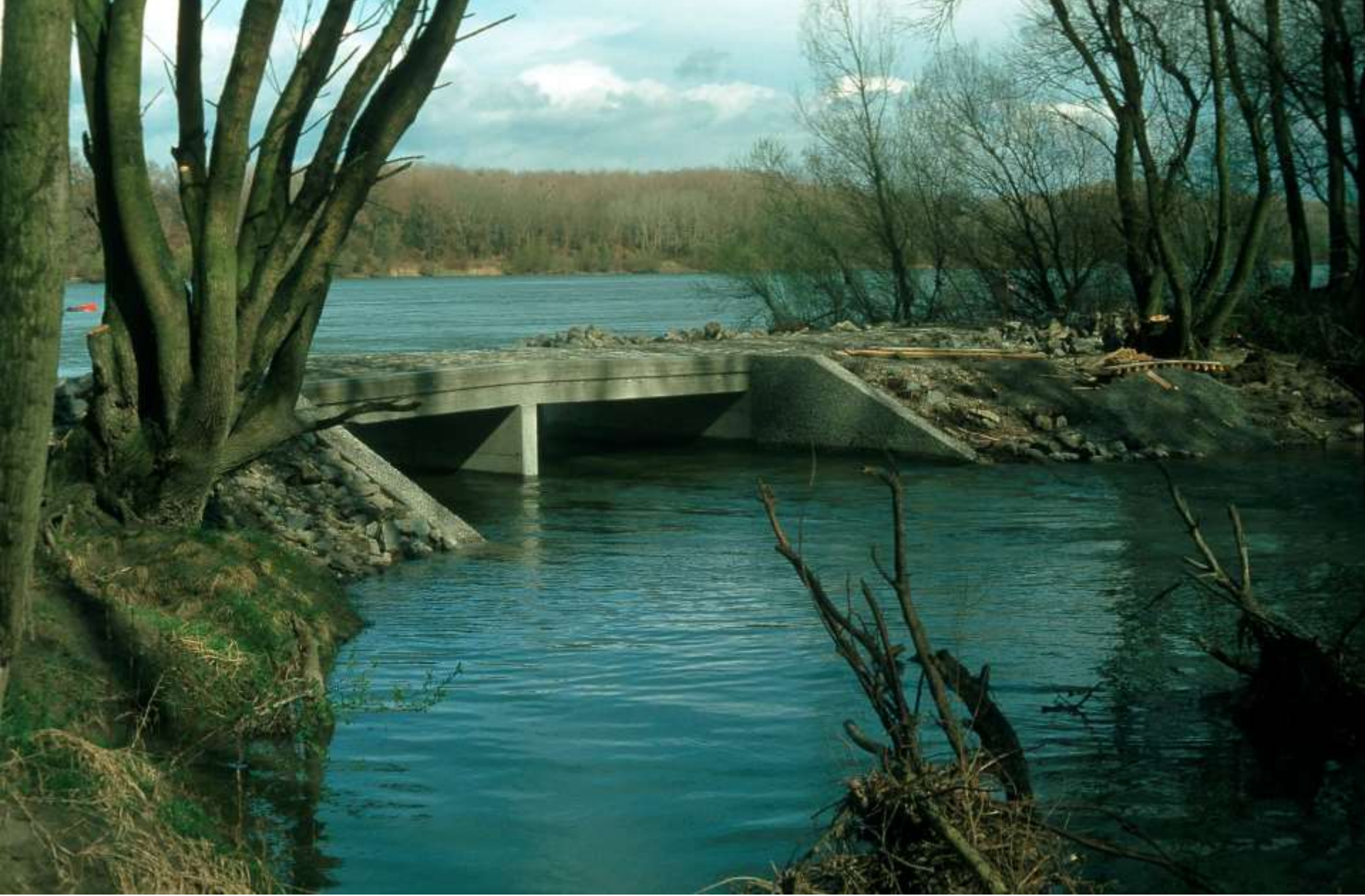
Inflow area Haslau, culvert
